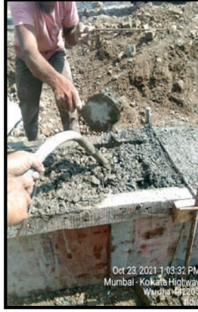
Plinth/Ground Beam Concreting
