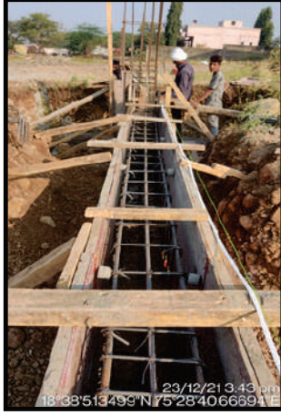
Ground beam Reinforcement & Shuttering
